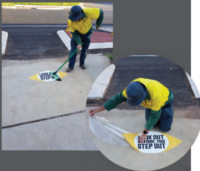
Photo: Installation of 'Look out before you step out' stickers.
