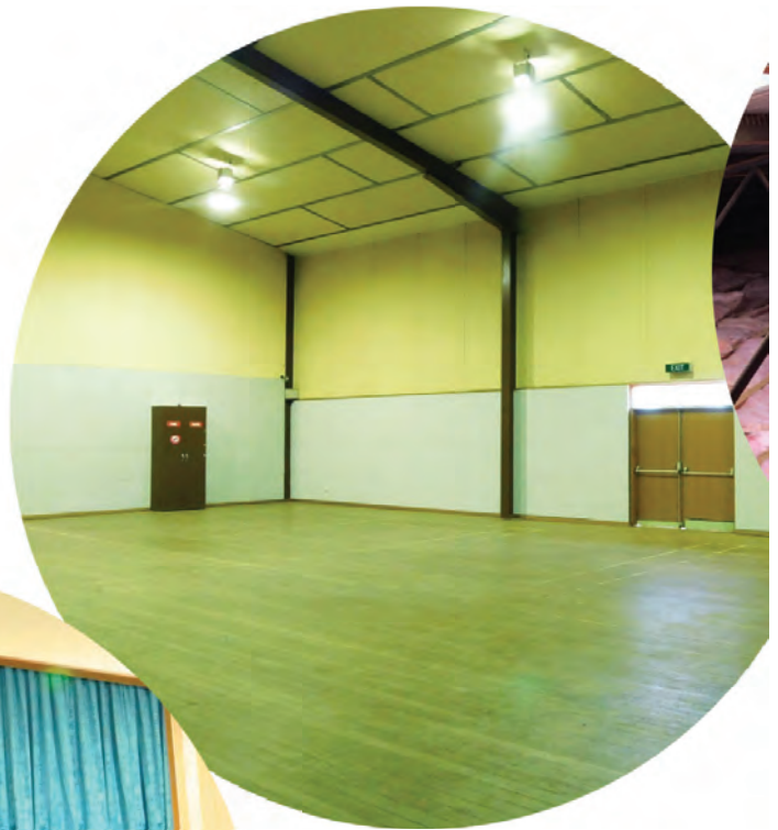
Photo right: New ceiling soundproofing installed at the Barellan Community Hall.
