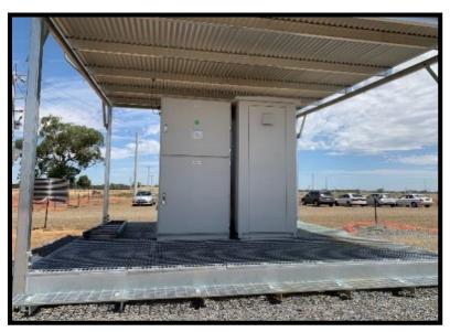
Figure 19 Typical HV switchboard and platform (Source: ACEnergy)
