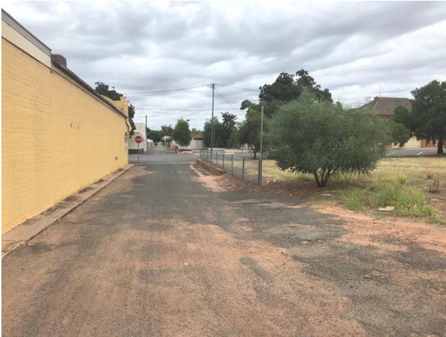
Photo 9: view of retaining wall & fence at Watkins Lane
