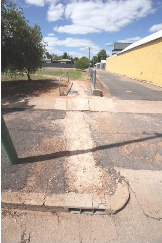
Photo 15: view of East St stormwater discharge
