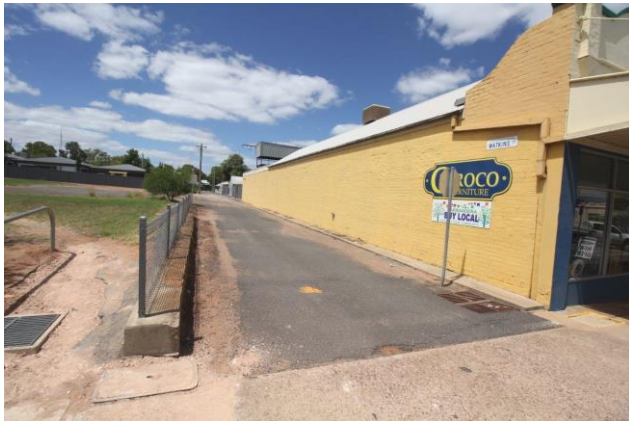
Photo 5: view of retaining wall at Watkins Lane
