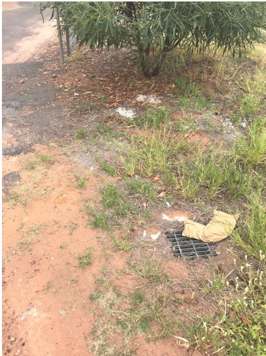
Photo 17: view of site stormwater pit at Watkins Lane
