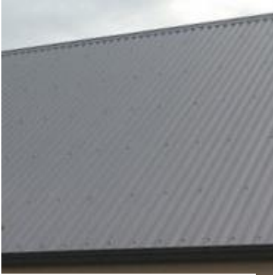
Roof – corrugated windspray + monument gutters
