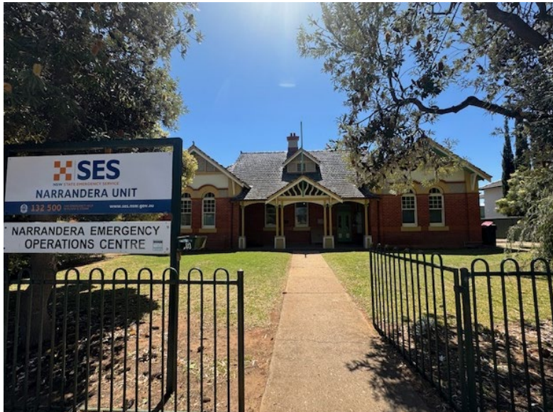
Narrandera Emergency Operations Centre located at 17-21 Twynam Street, Narrandera
