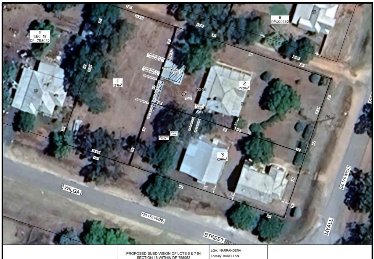
Figure 3 Close up Aerial Image of the development site and surrounds (Source: Rivland Surveyors)
