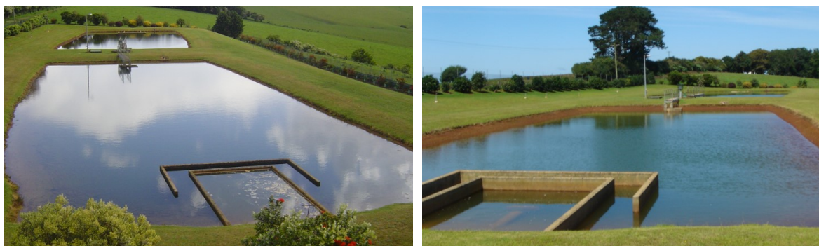
Appendix Figure A-6: Lagoon Sedimentation Clarifier
