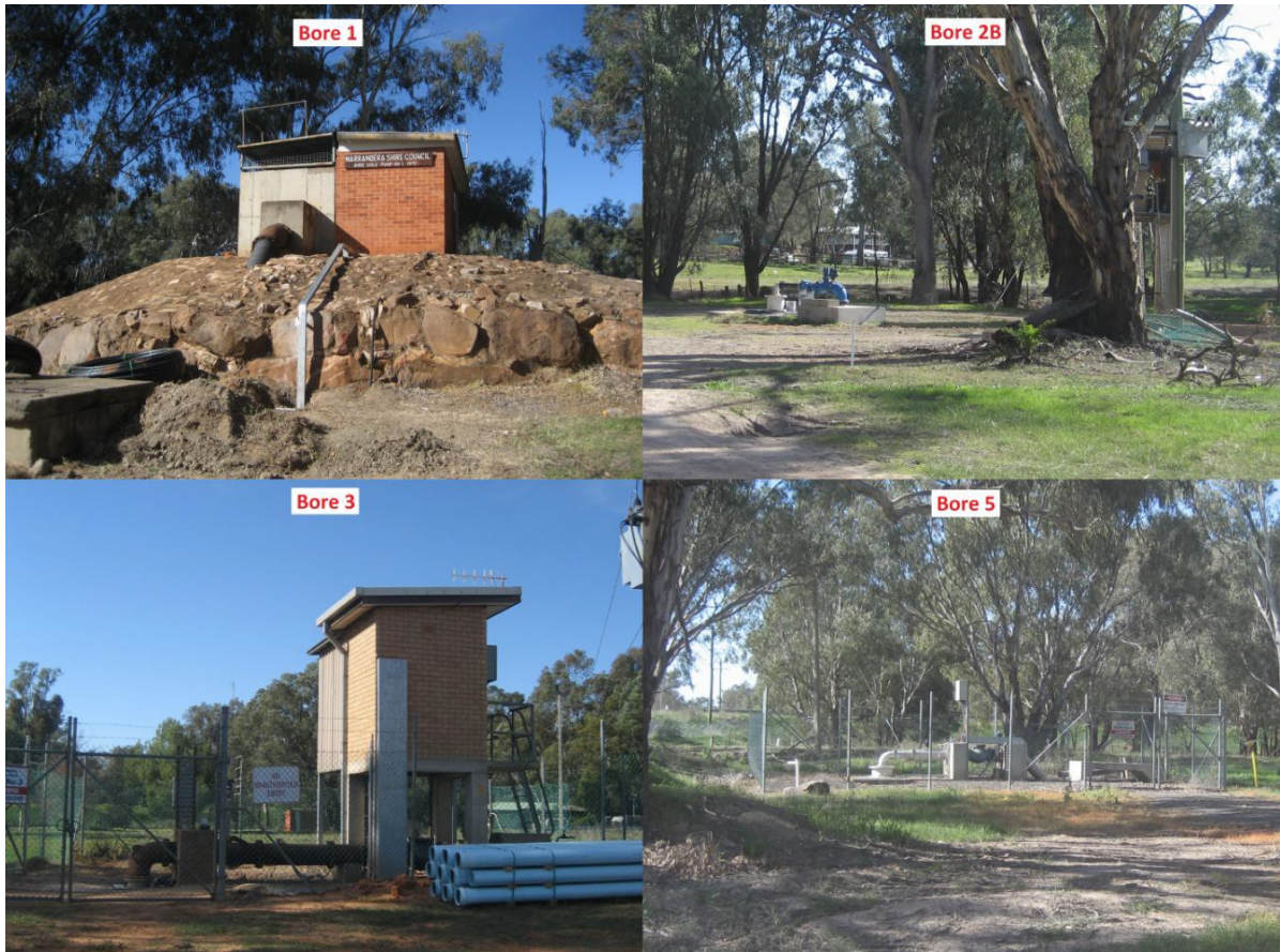
Figure 3-1: Images of bores (CWT, Narrandera Water Treatment Plant Audit Report, 2015)
