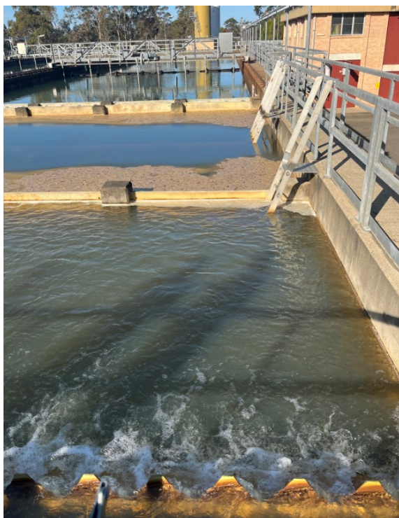
Appendix Figure A-3: Conventional horizontal flow sedimentation clarifier
