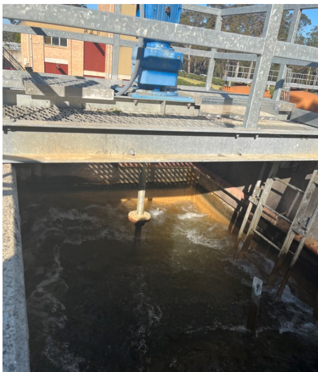
Appendix Figure A-2: Impeller flash mixer
